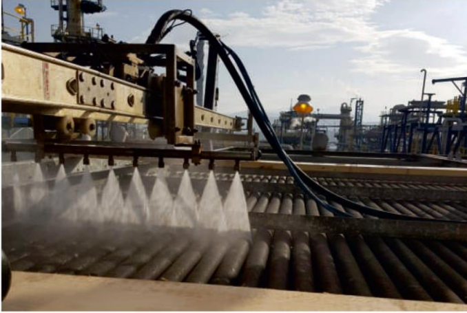
Cleaning of inside bundles and outside finned pipes. The cleaning system is easily adapted on the finned tubes surface by using special design coupling devices.
