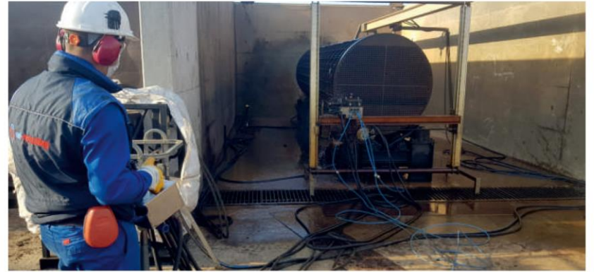
The cleaning operations are performed in-situ by using modular, portable, safe and easy to assemble modules.
