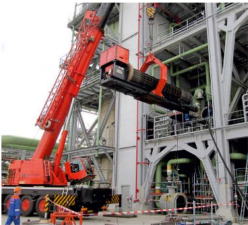
We use bundle extractors to eliminate the risk of damage.
