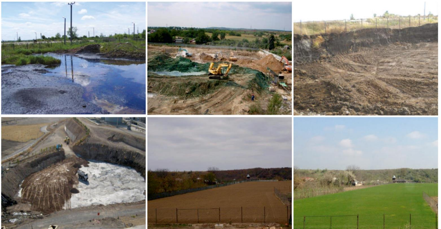
Overview of the operation for a contaminated site with hydrocarbons
